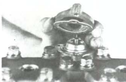
Fig. 35—Installing outlet elbow.
